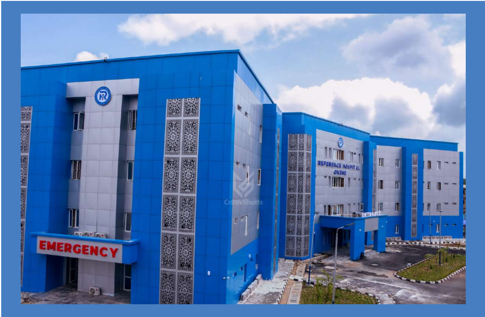
Side view of the Reference Hospital, Okene
