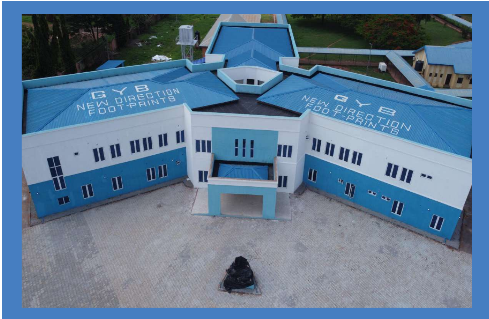
Front view of one of the newly Completed Ultra-Modern Hospitals
